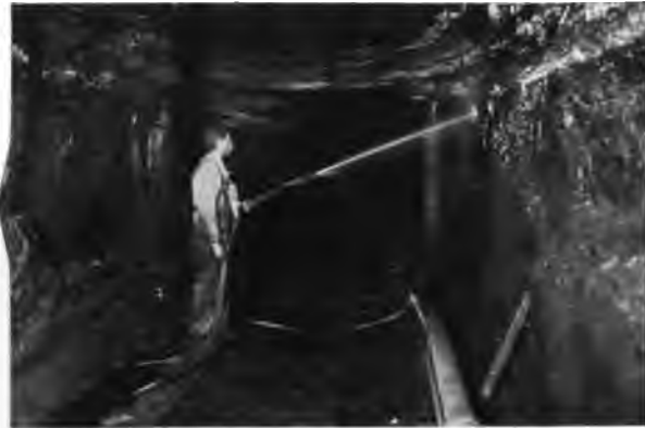
Fig. 3. Water Connection for Washing Down Dust.*
